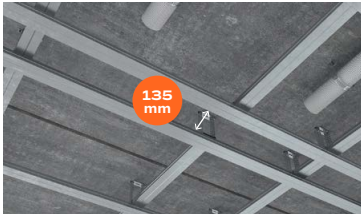
Installation width between profiles: 135 mm / ≈ 5,31".
