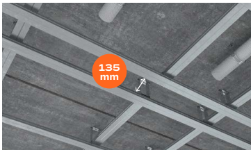
Installation width between profiles: 135 mm / ≈ 5,31".
